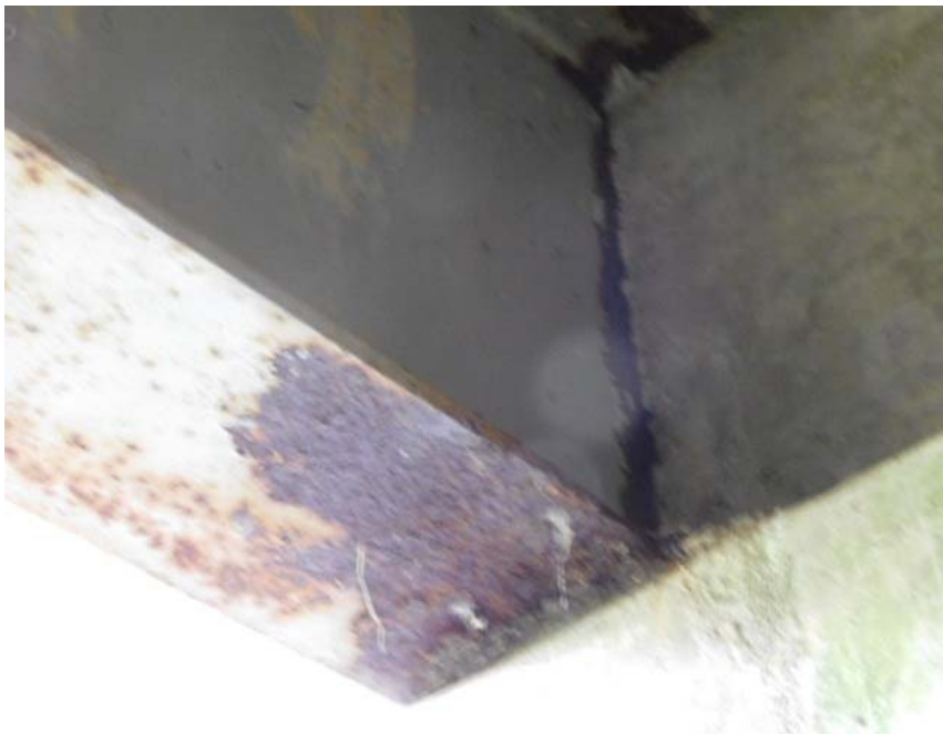
SPAN # 1 STEEL I BEAM "A" HEAVY CORROSION
