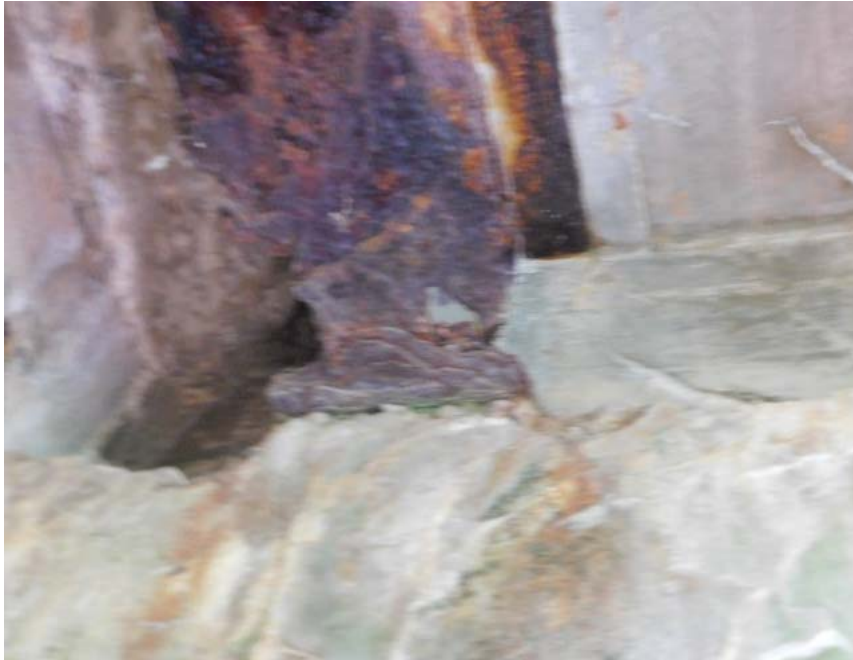
SPAN # 1 STEEL I BEAM "H" SECTION LOSS
