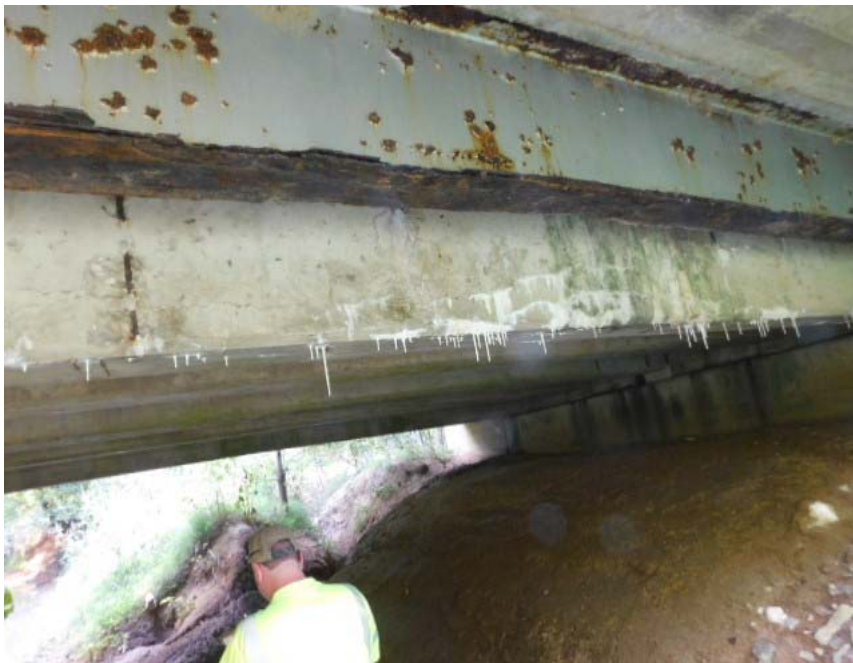
SPAN # 1 GIRDER "C" SPALLING TO STEEL & CRACKING
