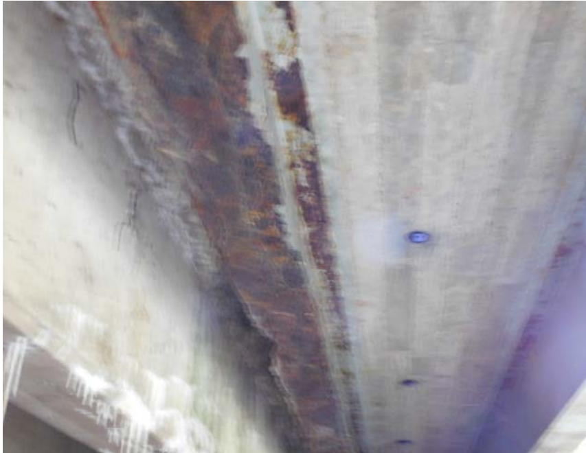
SPAN # 1 STEEL I BEAM "B" SECTION LOSS
