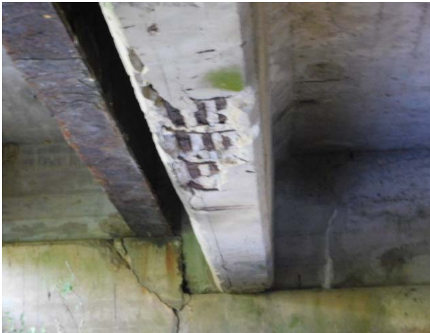
SPAN # 2 GIRDER "C" SPALLED TO STEEL
