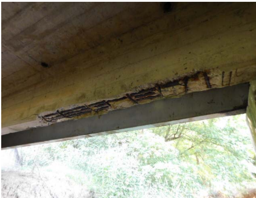
SPAN # 2 GIRDER "G" SPALLED TO STEEL
