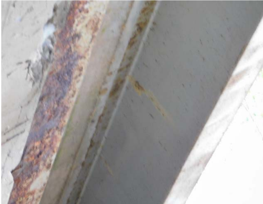
SPAN # 2 STEEL I BEAM "H" HEAVY CORROSION
